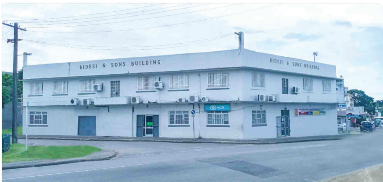
Bidesi & Sons Building, Waimanu Rd, Suva.
